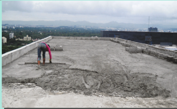
Light weight concrete being laid on a terrace slab.
